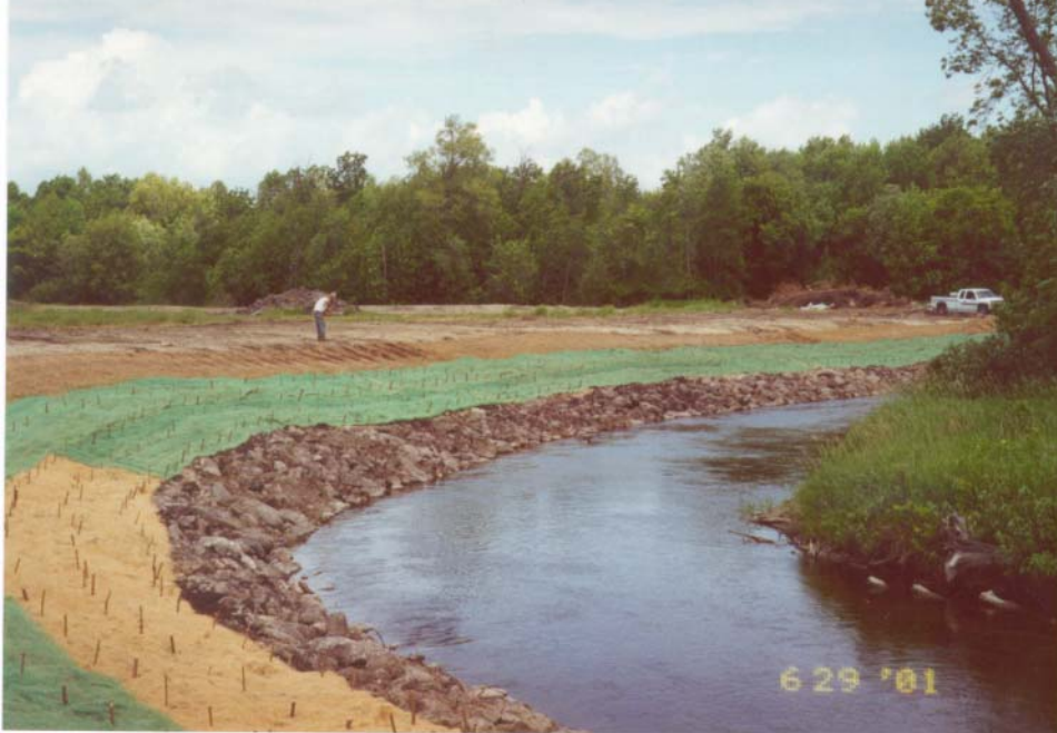
Bank stabilization site after completion of construction.
