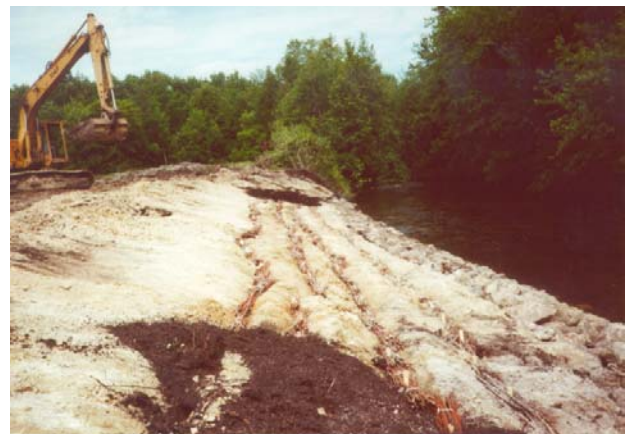
Installation of willow stakes and bundles at the Greenwood 27 site.
